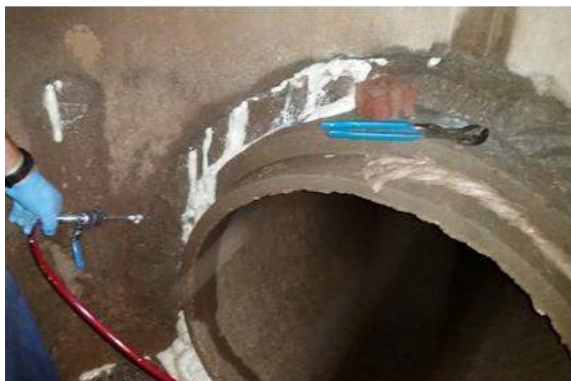
Pressure chemical grouting
