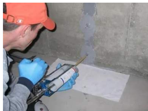
Chemical grouting with cartridge gun
