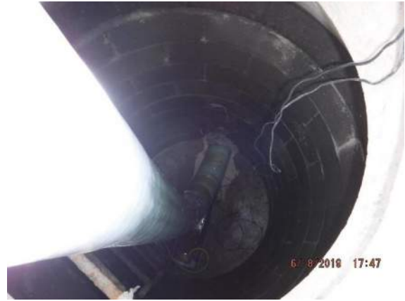
Hot water cured CIPP
