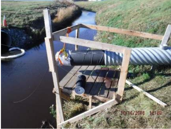
Curing UV CIPP liner
