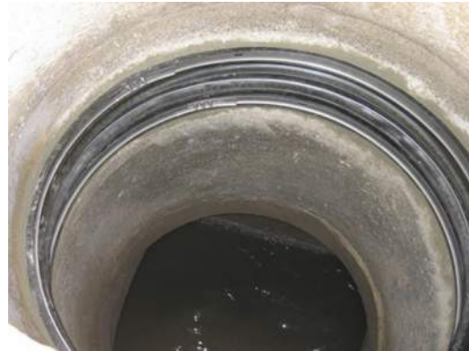
Cretex Internal Pipe Joint Seal
