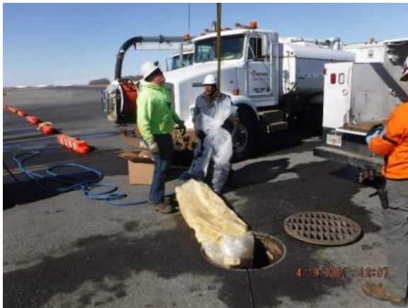
Install into pipe and pull into place
