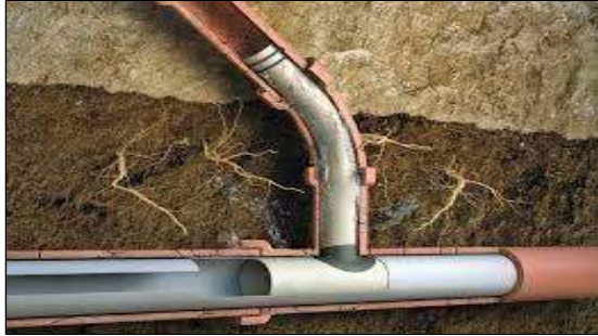
T-liner system at the sewer main
