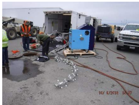
Equipment for UV cured CIPP
