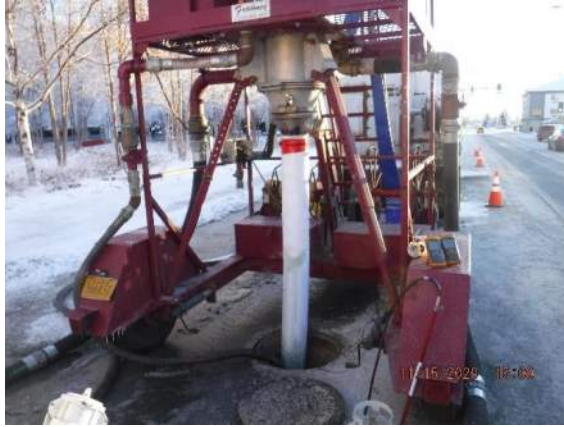
Hot water cured CIPP
