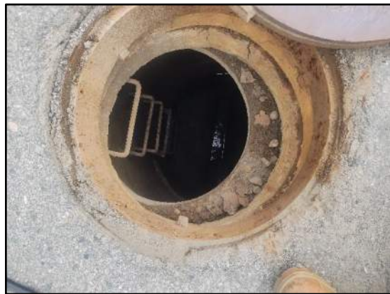
MH 19-0031, cone and chimney offset
