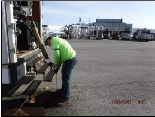
CCTV Camera Truck in Operation
