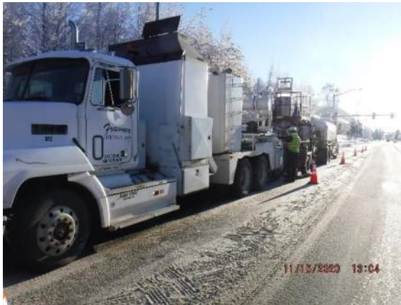
Equipment required for hot water CIPP
