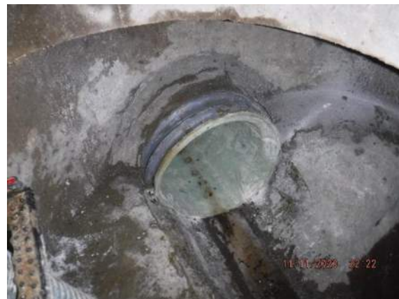
Hot water cured CIPP complete
