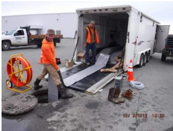
Pulling UV cured CIPP into place
