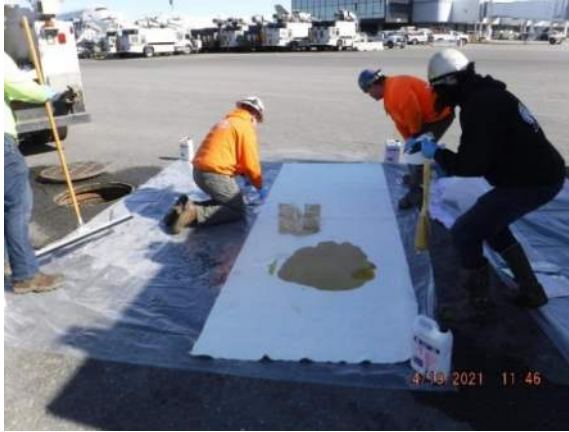
Resin installed over fiberglass matt
