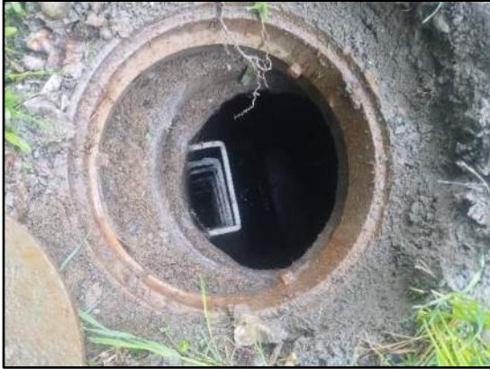
MH 19-0027, frame-chimney offset
