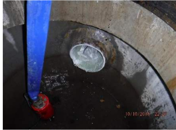
UV cured CIPP liner complete
