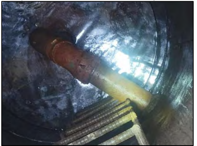
Image 6 – Elevated Southeast 6" Influent Pipe
