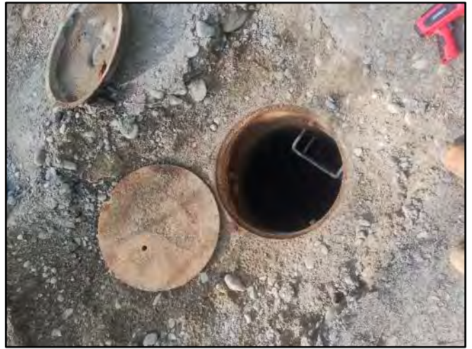
Image 2 – Frame, Catchpan and Cover
