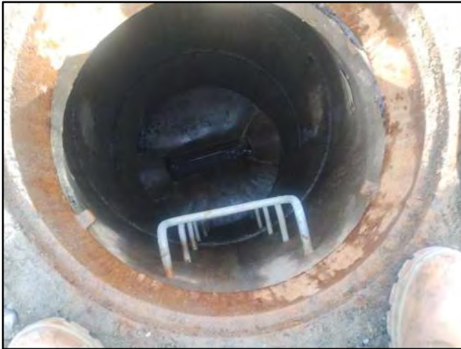
Image 3 –Frame, Cone, Barrels, and Steps
