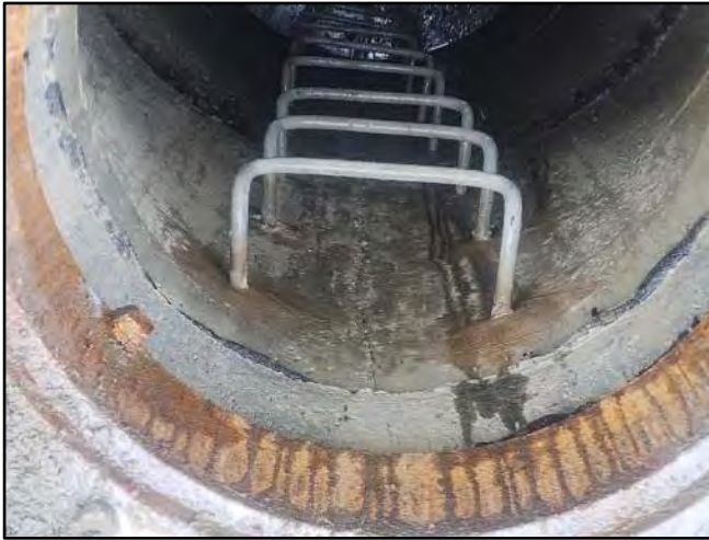
Image 3 – Chimney, Cone, and Stairs
