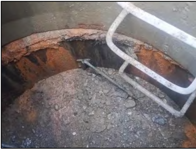
Image 3 – Cone and Base Offset
