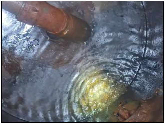
Image 4 – North Connection with Massive Submerged Gusher
