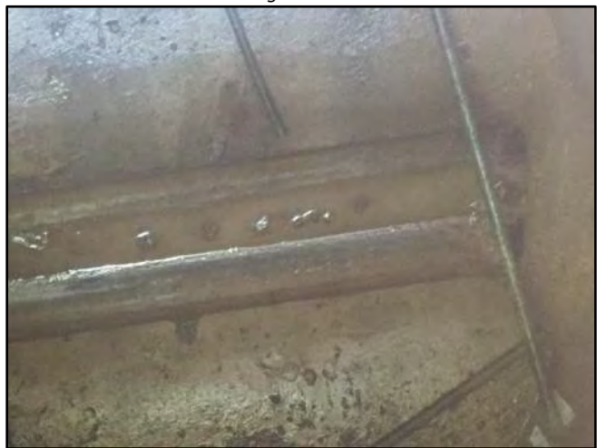
Image 6 – North Effluent Connection
