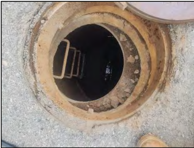
Image 3 – Chimney and Cone Offset
