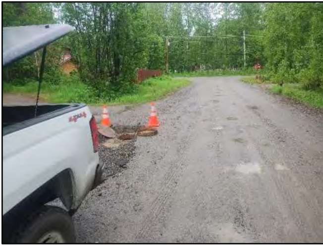
Image 1 – MH facing North towards intersection
