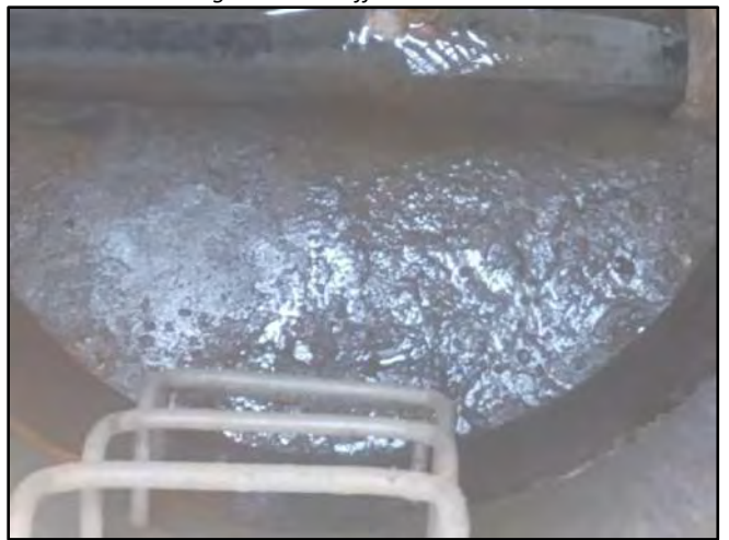
Image 6 – Standing Water on Shelf
