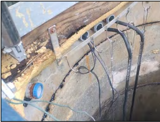
Image 3 – Wooden Studs & Spray Foam Insulation
