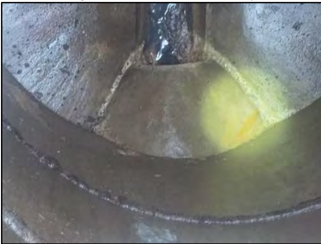
Image 5 – North Influent Connection
