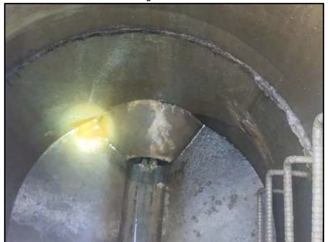
Image 6 – I&I runner along East Side, Mineralization
