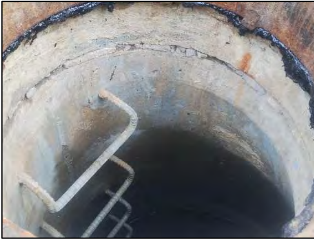
Image 3 – Chimney and Cone
