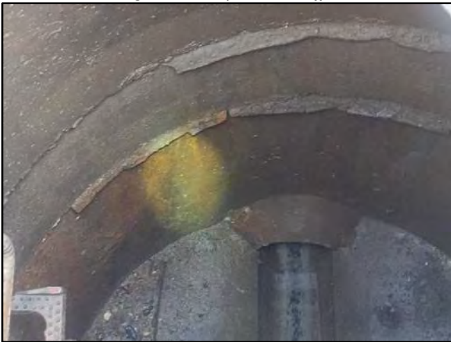
Image 5 – Mineralization and Influent Connection
