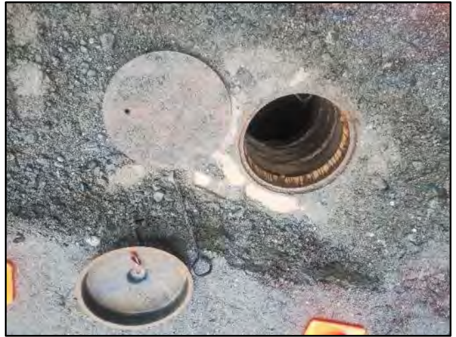
Image 2 – Frame, Cover, and Catchpan
