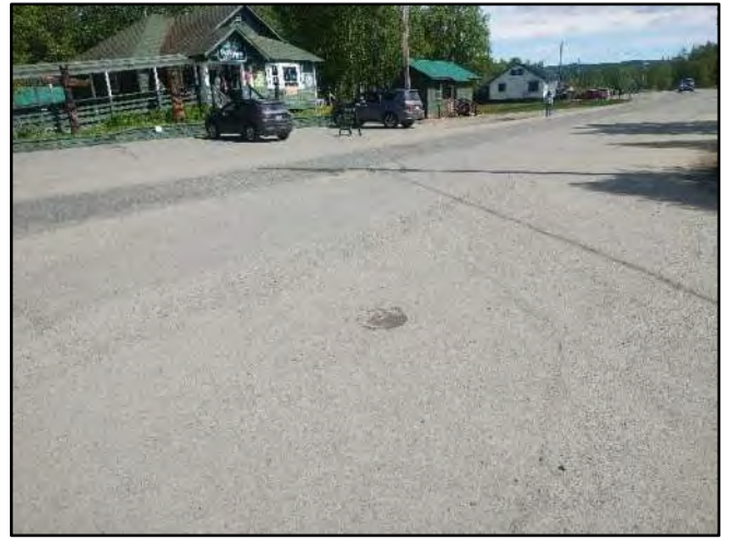
Image 2 – CO Facing East
