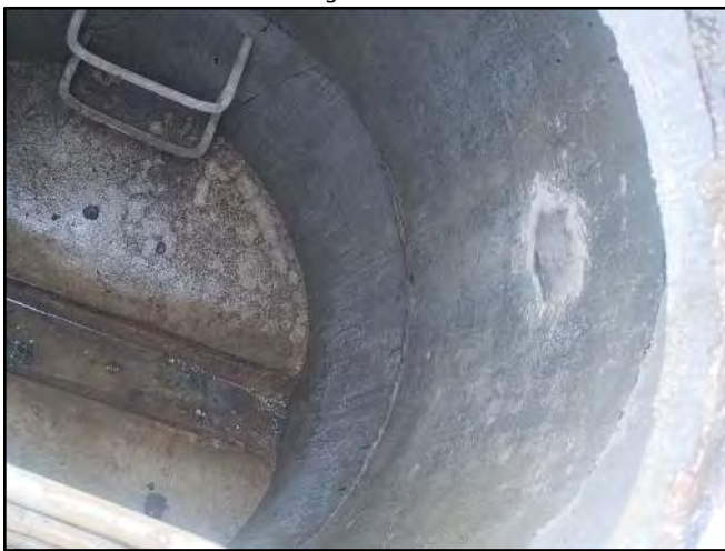
Image 5 – Base and Barrel
