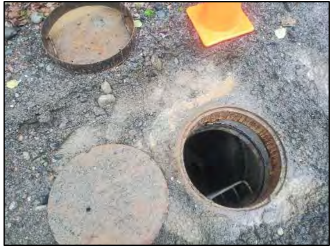
Image 2 – Frame, Catchpan and Cover
