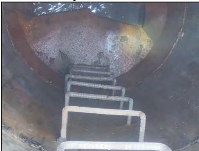
Image 5 – Dripper along North Connection
