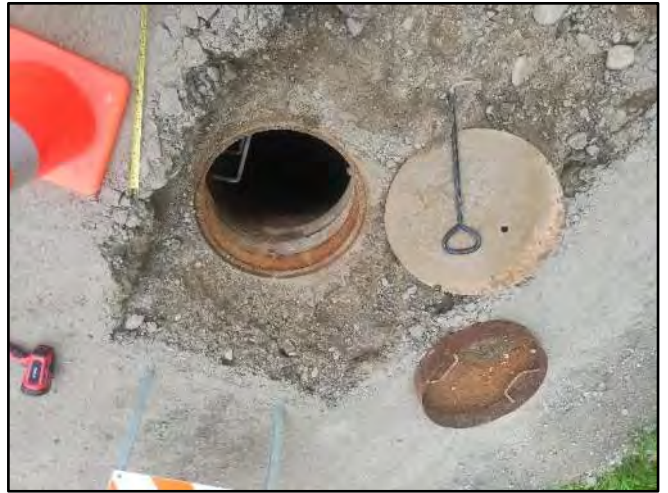
Image 2 – Frame, Cover, and Catchpan
