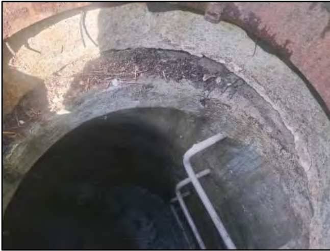
Image 3 – Chimney and Cone Offset
