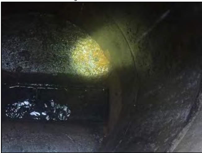
Image 5 – Mineralization and Dripper near Influent Connection
