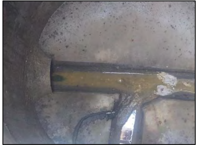
Image 4 – East Influent Connection
