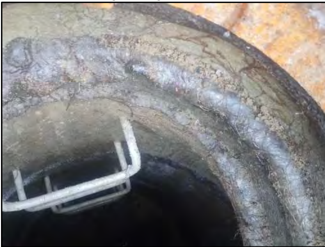
Image 5 – Root Intrusion along Chimney
