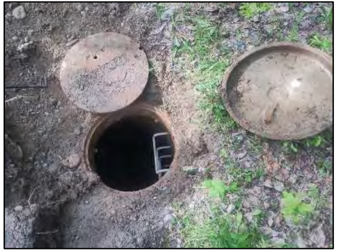
Image 2 – Frame, Catchpan and Cover
