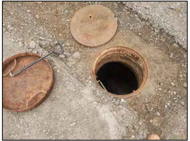
Image 2 – Frame, Catchpan and Cover
