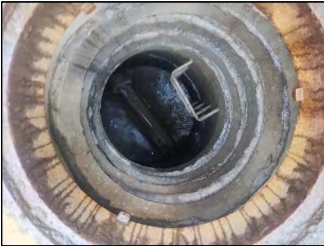
Image 3 – Frame, Chimney, and Cone
