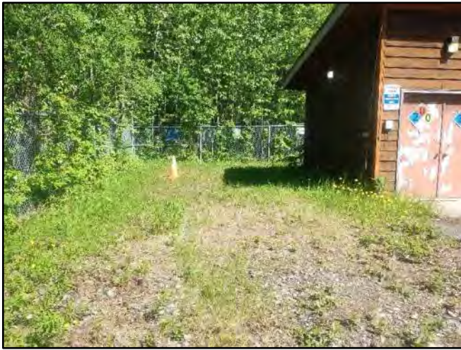
Image 1 – CO Facing North towards Chemical Storage
