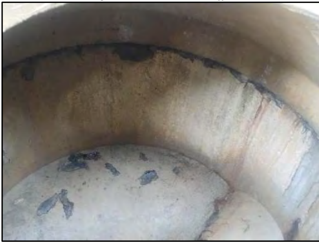
Image 5 – Mineralization from Cone/Base Joint
