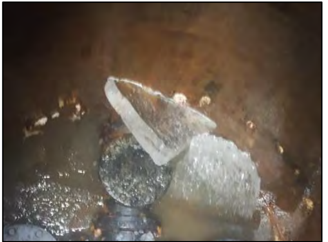
Image 4 – North Connection and Ice Chunks
