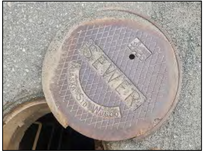
Image 2 – Cover and Frame Attached
