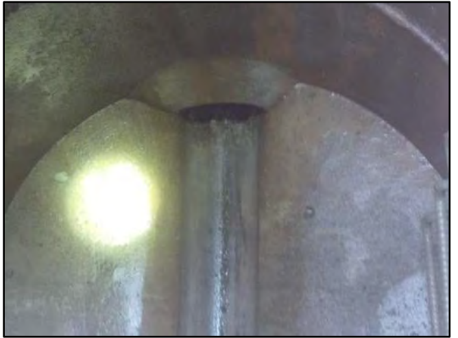
Image 4 – South Effluent Connection
