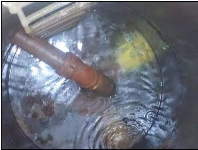
Image 5 – West Effluent Connection
