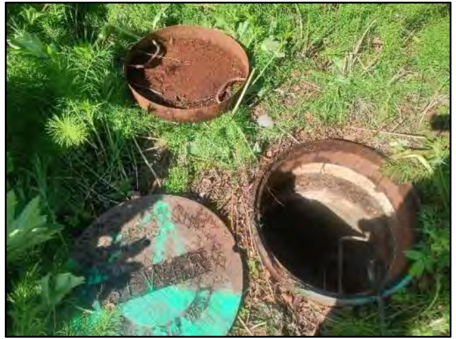
Image 2 – Cover, Catchpan, and Frame
