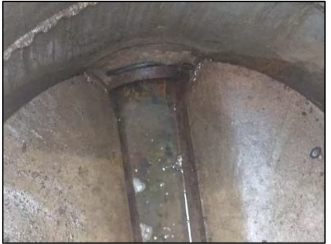
Image 4 – South Effluent Connection
