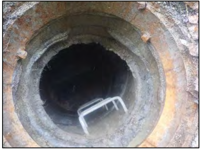
Image 2 – Frame, Chimney, and Stairs
