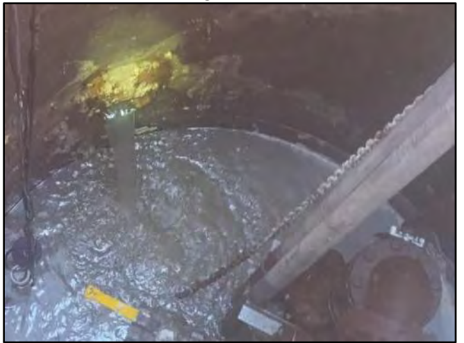
Image 6 – East Influent Connection
