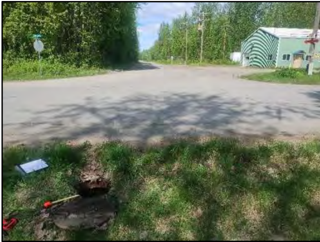
Image 1 – MH facing North on G St
