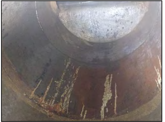
Image 4 – Mineralization from Barrel/Barrel Joint
