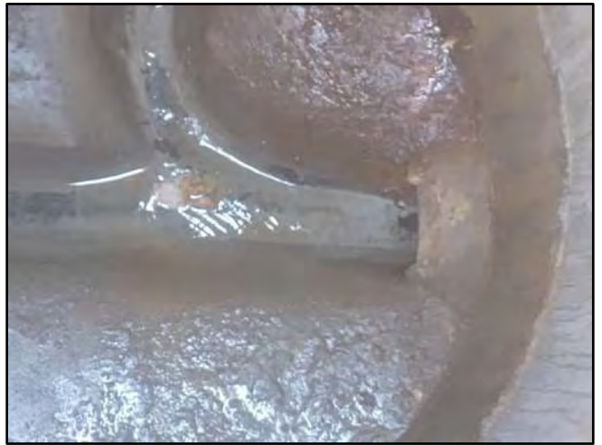
Image 4 – West Effluent Connection
