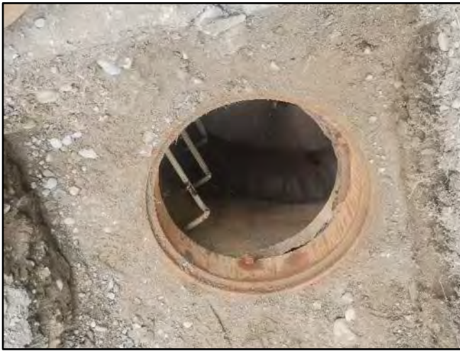
Image 3 – Frame and Cone Offset
