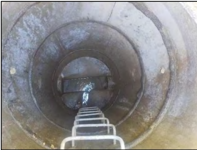
Image 3 – Cone, Barrels, and Base
