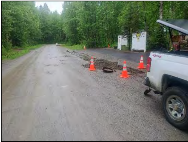
Image 1 – MH facing South along H St
