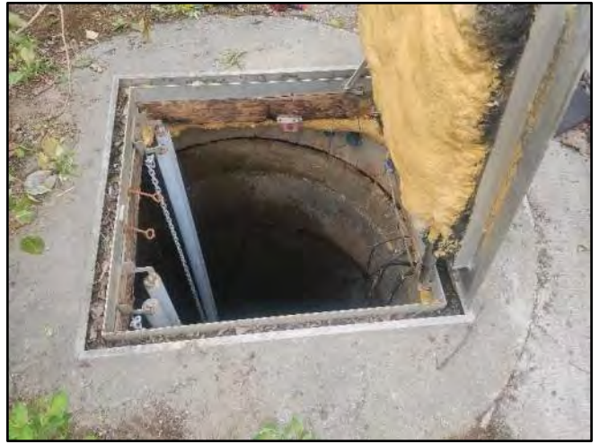
Image 2 – Cover, Frame, and Chimney
