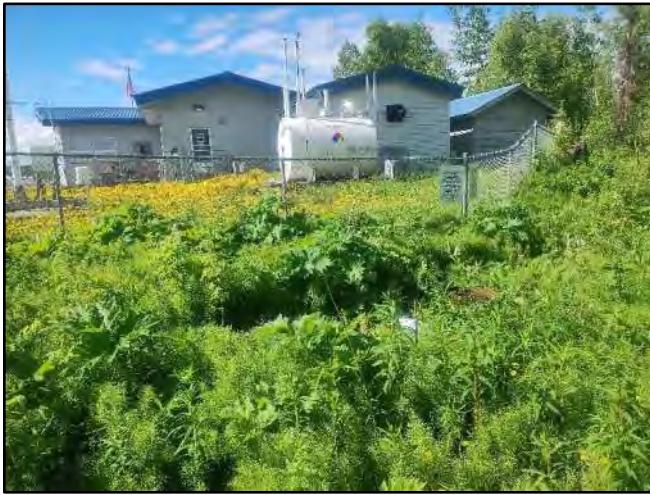
Image 1 – MH facing South to FAA Facility
