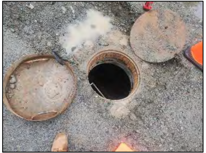
Image 2 – Frame, Catchpan and Cover
