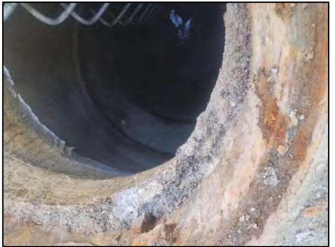
Image 4 – Root Intrusion along Cone
