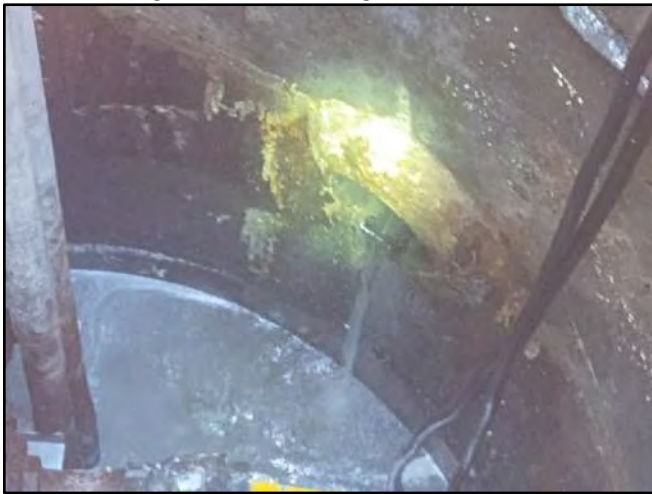
Image 5 – West Influent Connection
