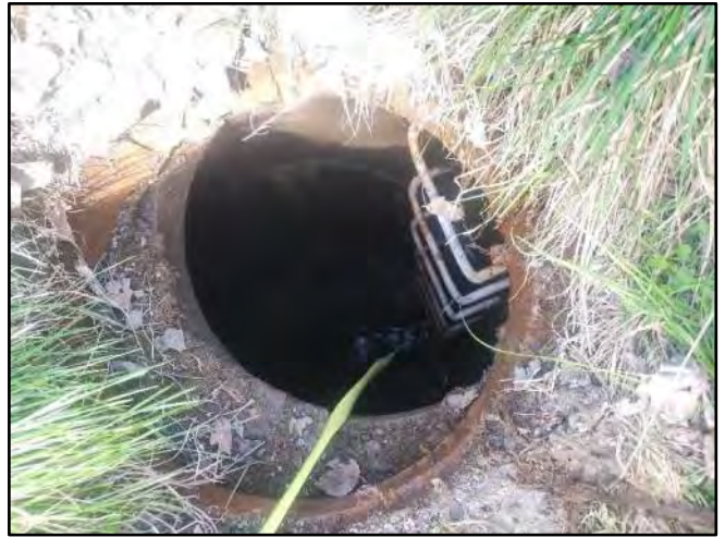
Image 2 – Frame and Cone Offset
