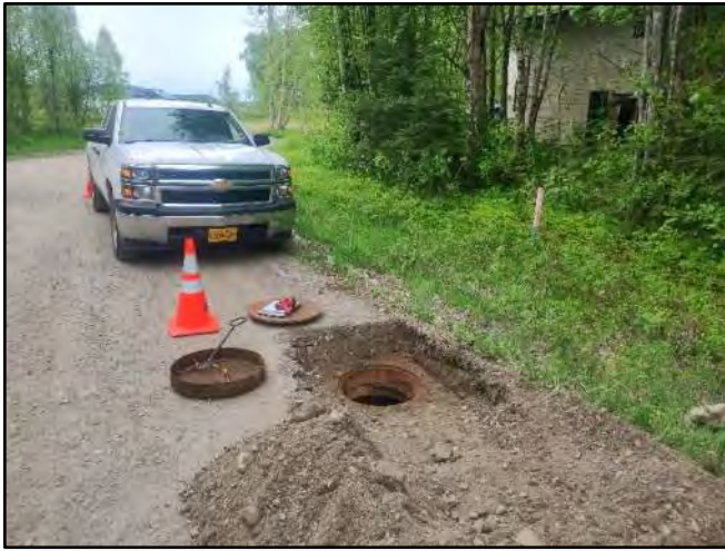
Image 1 – MH facing South towards curve
