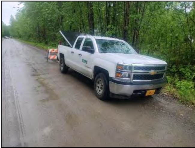
Image 1 – MH facing South along H St
