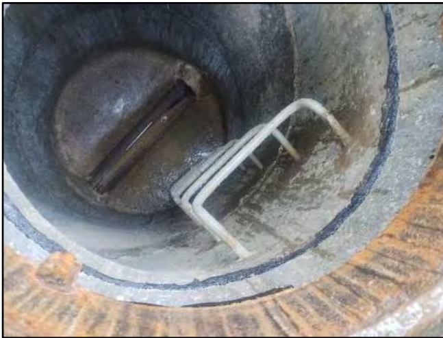
Image 3 – Chimney, Cone, and Stairs
