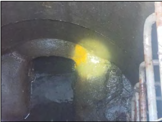
Image 5 – West Effluent Connection and Stairs
