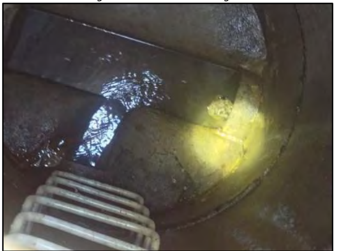
Image 6 – I&I Dripper and North Effluent Connection
