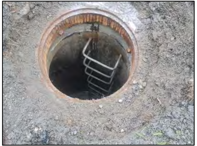
Image 2 – Frame and Chimney
