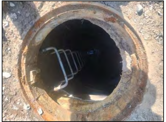
Image 2 – Frame & Cone, Offset and Root Intrusion
