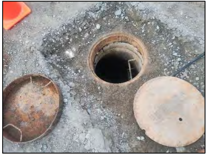
Image 2 – Frame, Catchpan and Cover
