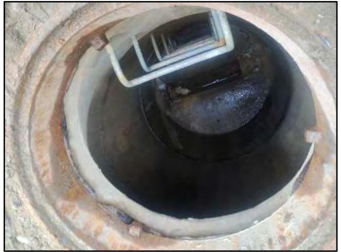
Image 2 – Frame, Stairs and Cone
