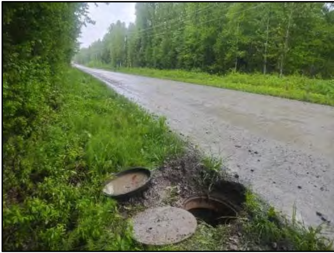
Image 1 – MH facing North on G St
