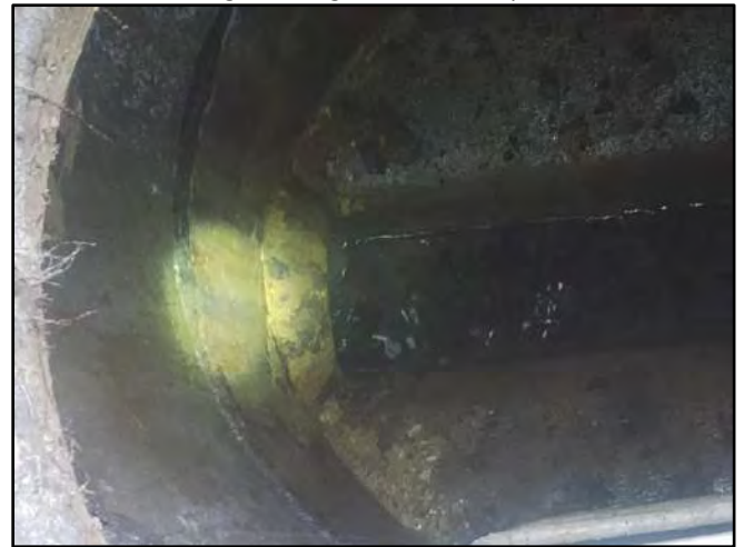
Image 6 – Mineralization from Barrel/Base Joint
