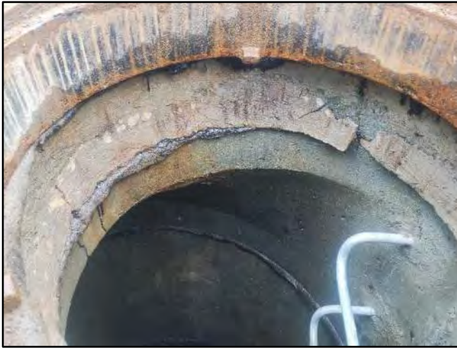
Image 3 – Chimney Cracking
