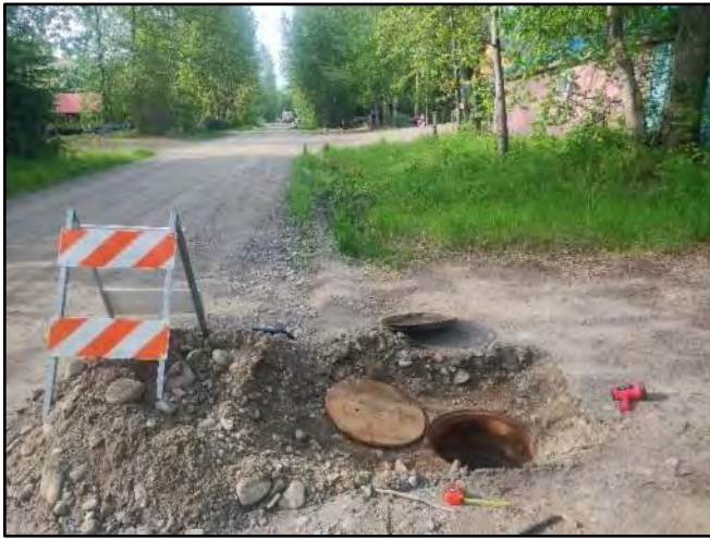
Image 1 – MH facing South along I St
