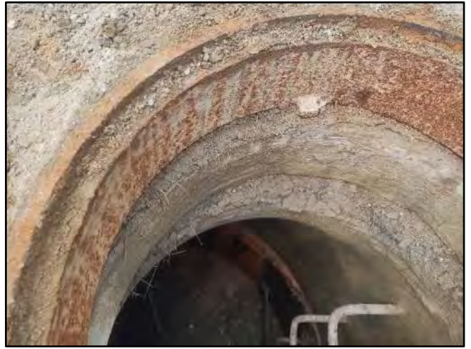
Image 2 – Frame, Chimney, and Cone Offset
