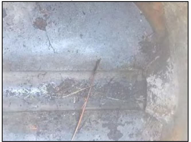
Image 6 – West Effluent Connection
