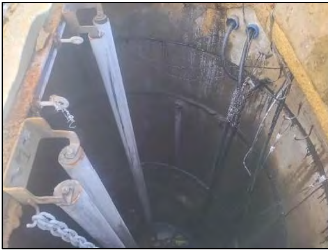
Image 3 – Frame, Reducing Slab, and Barrels
