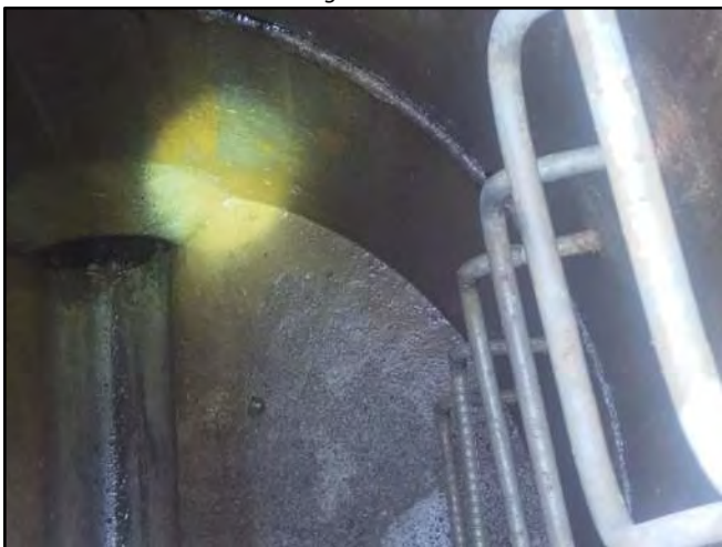
Image 5 – Mineralization
