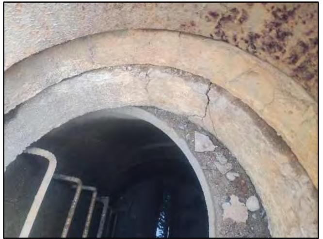
Image 4 – Chimney Cracking
