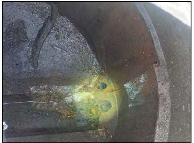
Image 6 – I&I Mineralization and Effluent Connection
