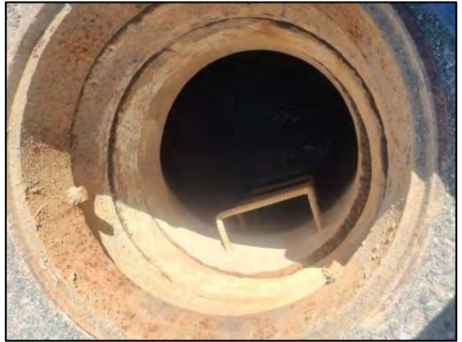
Image 2 – Frame and Chimney
