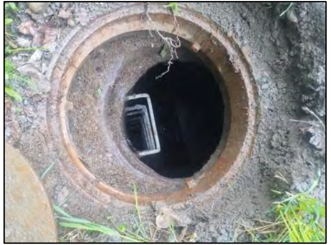
Image 2 – Frame, Chimney, and Cone Offset
