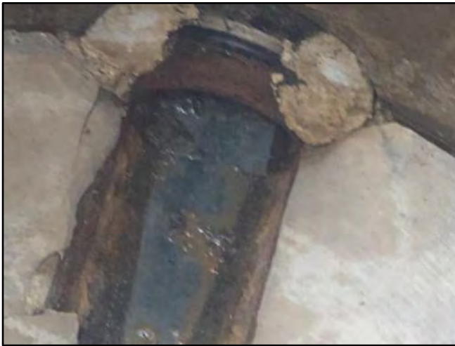
Image 3 – North Influent Connection
