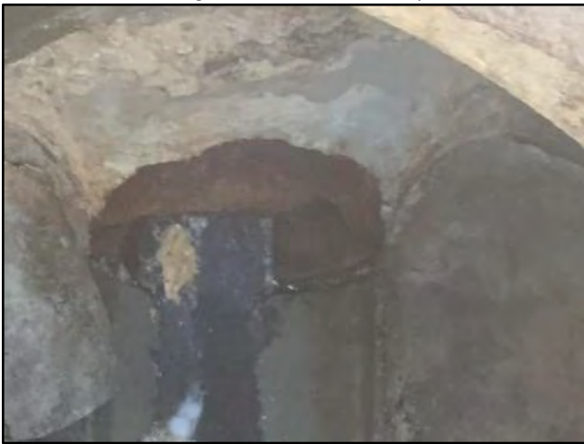
Image 5 – West Effluent Connection
