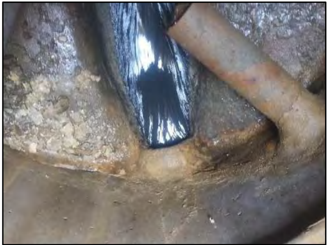
Image 4 – West Influent Connection
