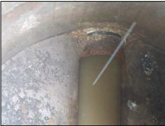
Image 5 – West Effluent Connection
