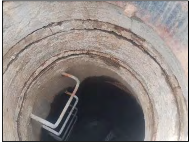
Image 4 – Chimney Cracking
