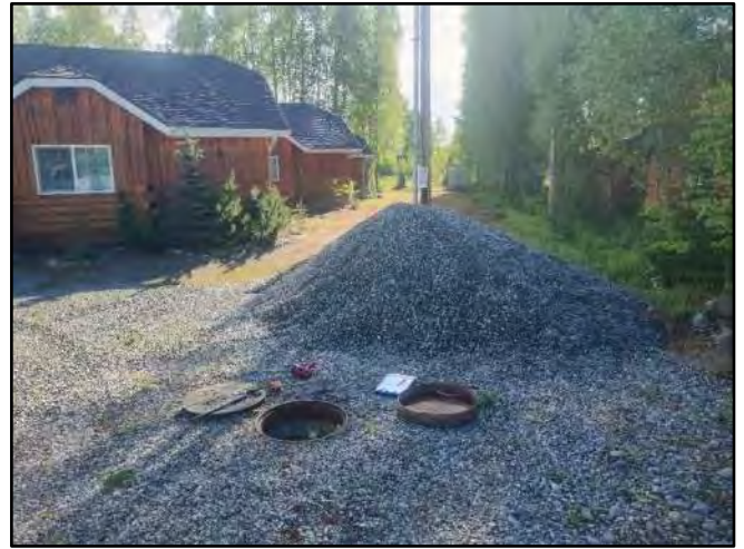
Image 2 – MH facing East toward Denali Fireside Cabins
