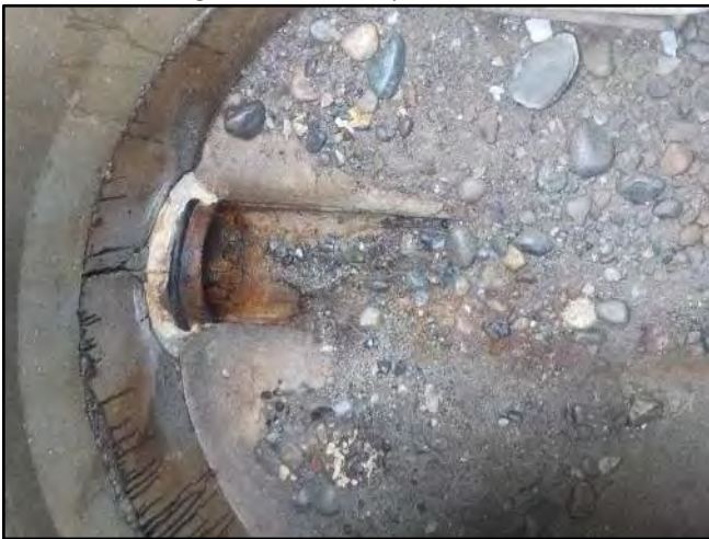
Image 5 – Sediment Build-up
