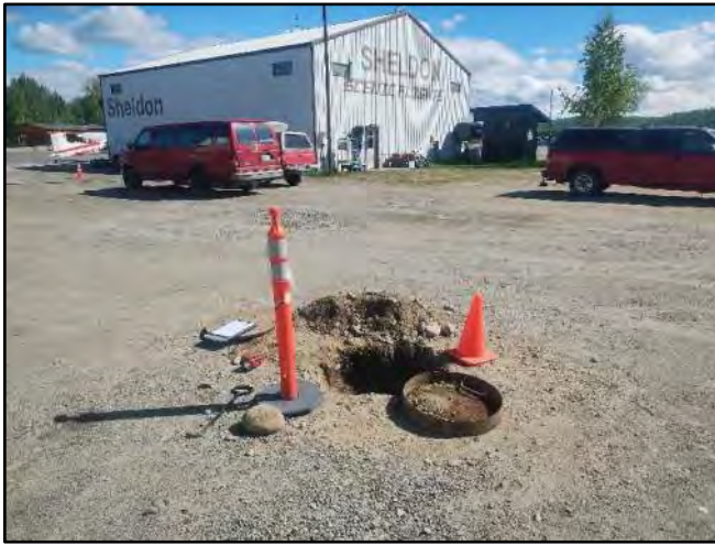
Image 1 – MH Facing Northeast
