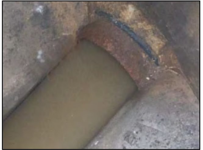
Image 4 – East Influent Connection
