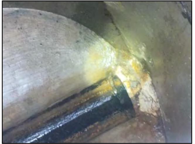
Image 4 – West Influent Connection
