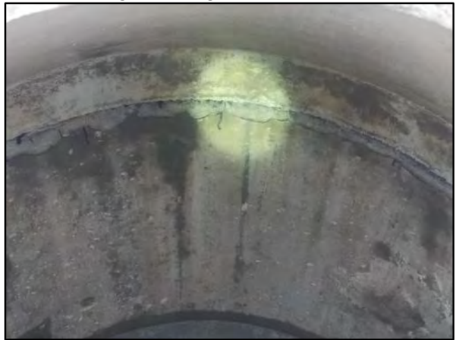
Image 6 – Cone/Base Joint
