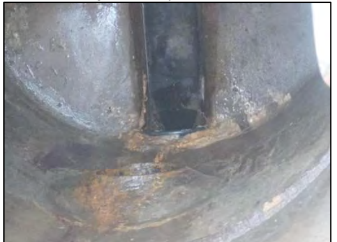
Image 6 – West Influent Connection
