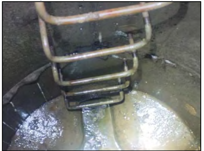
Image 6 – South Effluent Connection and Stairs
