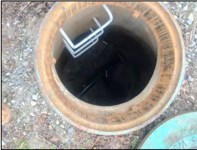
Image 3 – Frame, Cone, and Stairs
