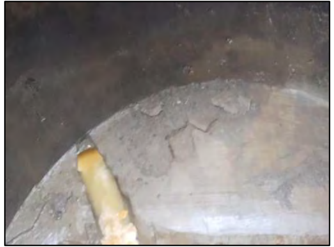
Image 4 – Sediment Build-up on Shelf
