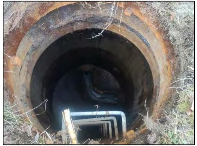
Image 2 – Frame, Chimney, and Steps
