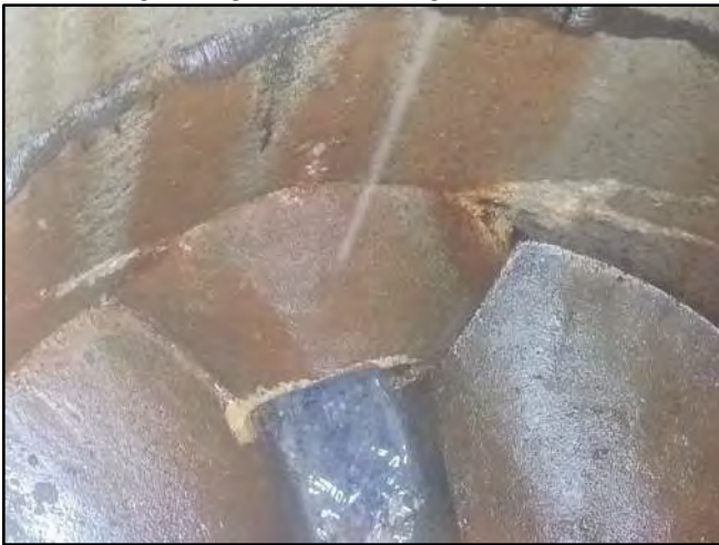
Image 5 – West Influent Connection
