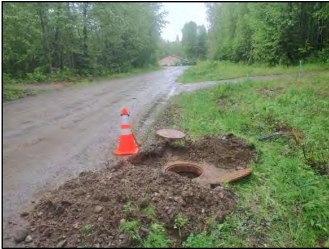
Image 1 – MH facing East on Main St
