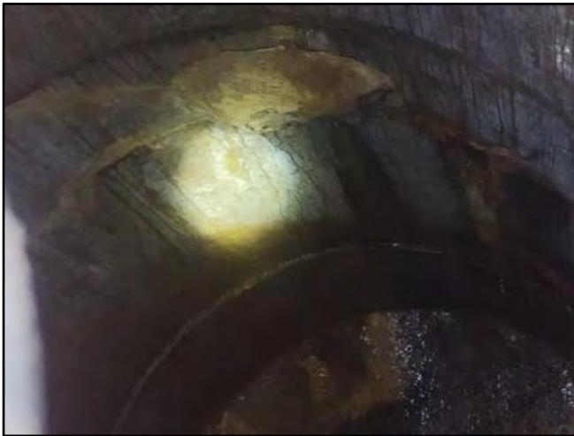
Image 3 – North Wall with Decommissioned Pipe
