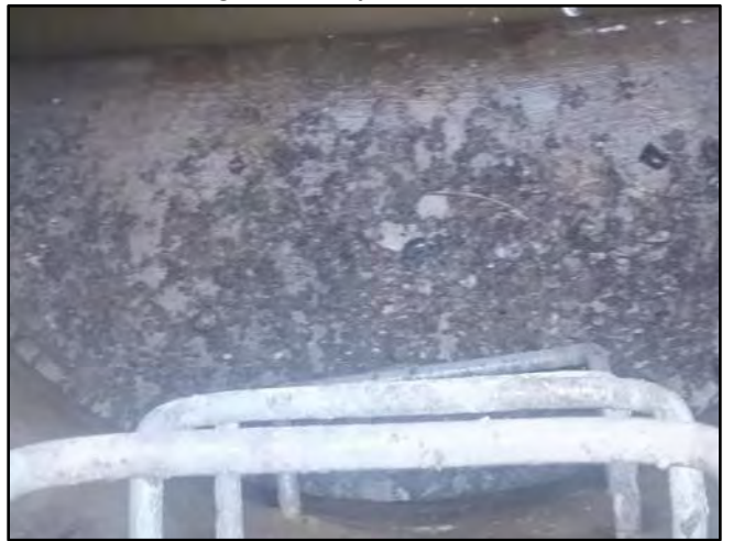
Image 6 – Sediment Build-up on Shelf
