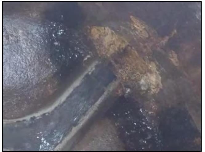
Image 6 – South Effluent Connection
