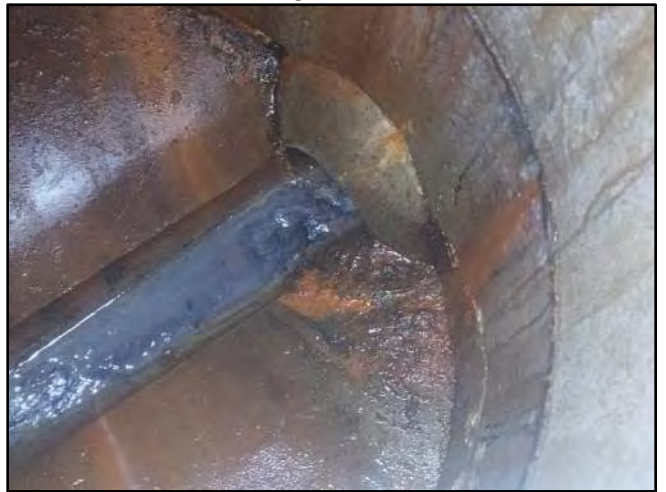
Image 6 – East Effluent Connection
