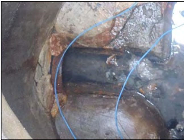
Image 3 – West Influent Connection
