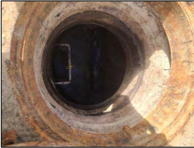
Image 3 – Frame and Chimney
