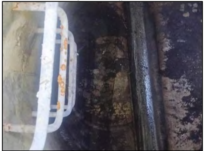
Image 6 – Stairs and Base
