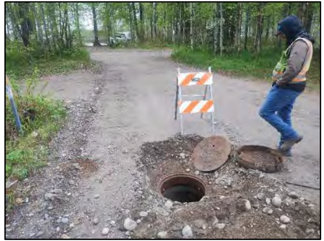
Image 2 – MH facing West along North Alley
