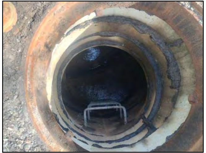
Image 2 – Frame, Chimney, and Steps
