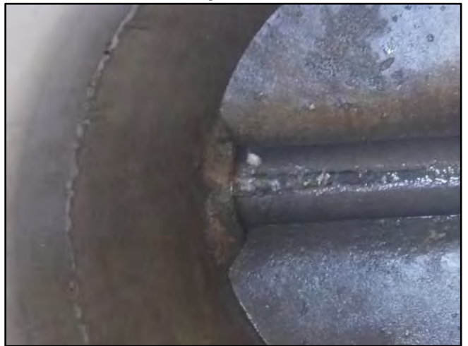
Image 6 – North Effluent Connection
