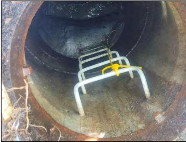
Image 3 – Frame, Cone and Stairs
