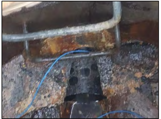
Image 4 – North Influent Connection
