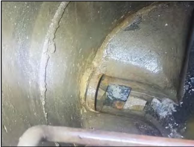
Image 3 – West Influent Connection
