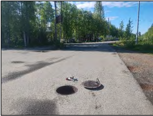
Image 1 – MH facing South in Parking Lot
