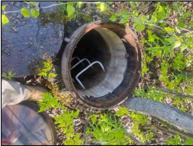
Image 3 – Frame, Chimney, and Cone
