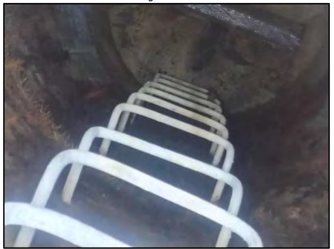
Image 6 – Root Growth along Barrel and Base
