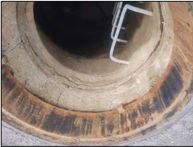
Image 3 – Frame and Chimney
