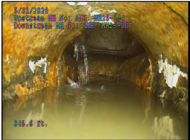
Image 5 – North Connection Gusher CCTV
