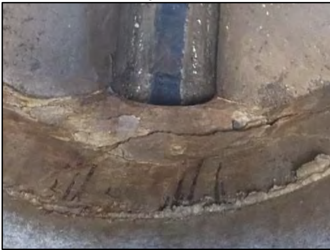
Image 5 – East Influent Connection
