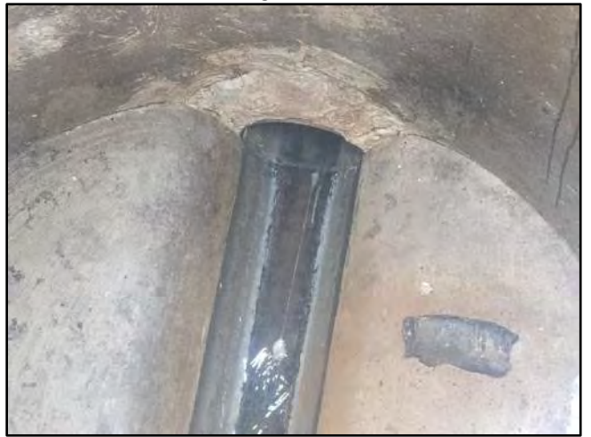
Image 6 – West Effluent Connection
