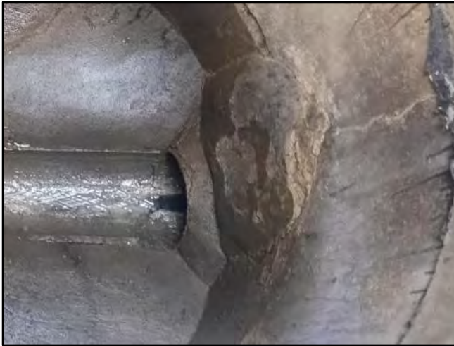
Image 3 – East Influent Connection
