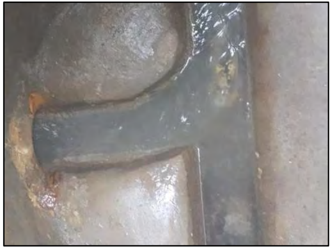
Image 4 – North Influent Connection
