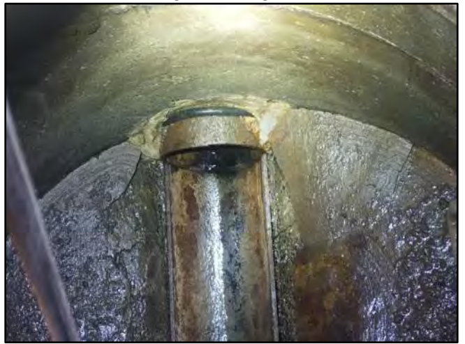
Image 6 – West Effluent Connection
