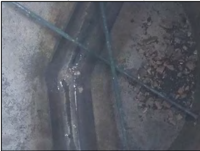
Image 5 – Sediment Build-up on West Shelf
