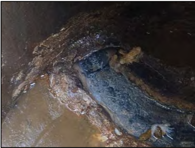
Image 5 – West Effluent Connection
