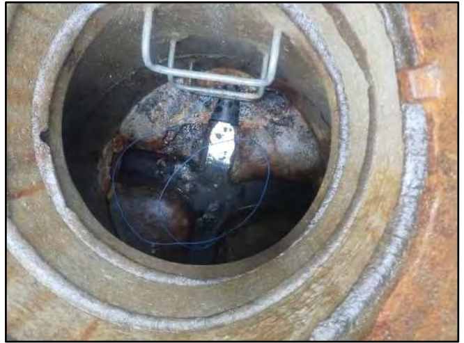
Image 2 – Frame, Chimney, and Stairs
