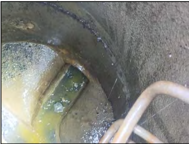
Image 5 – East Influent Connection
