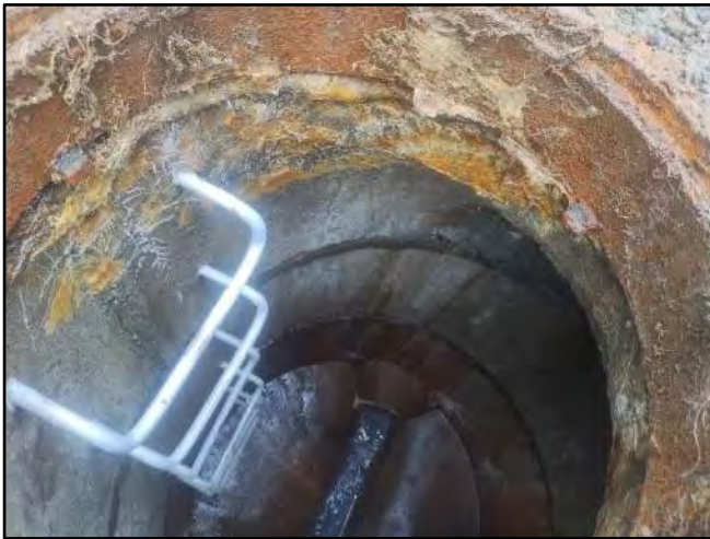
Image 3 –Organic Growth along Frame and Cone
