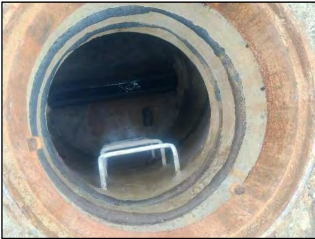
Image 3 – Chimney, Cone, and Stairs
