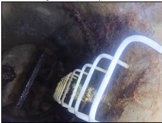
Image 5 – Root Growth on East Cone and Barrel
