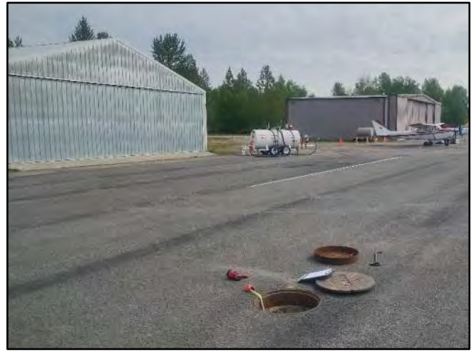
Image 2 – MH facing NE to Okonek Hangar
