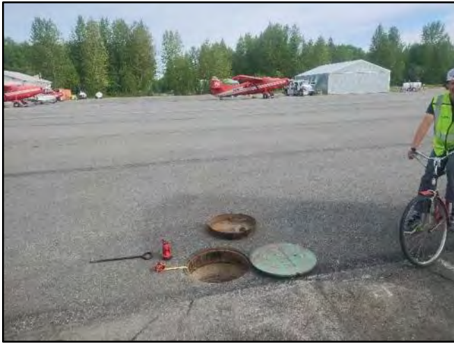
Image 1 – MH Facing North
