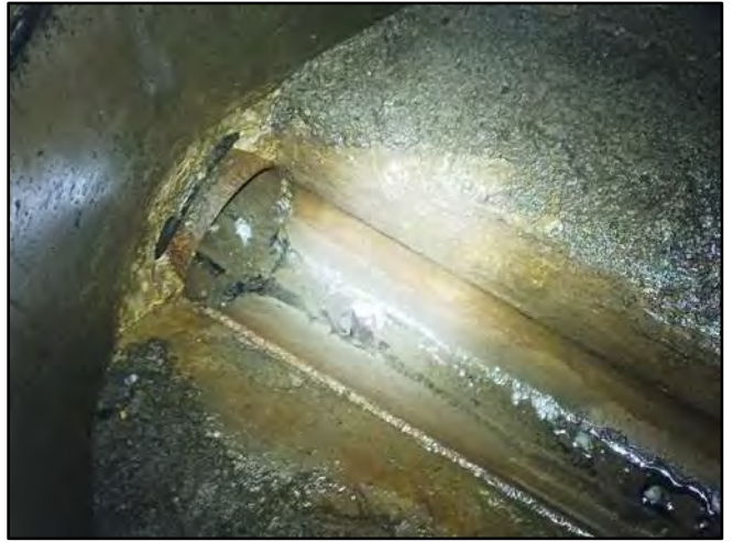
Image 4 – East Influent Connection
