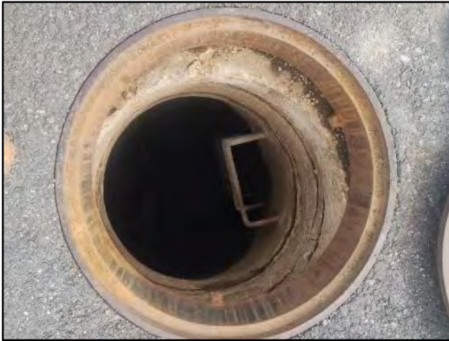
Image 3 – Frame and Chimney Offset
