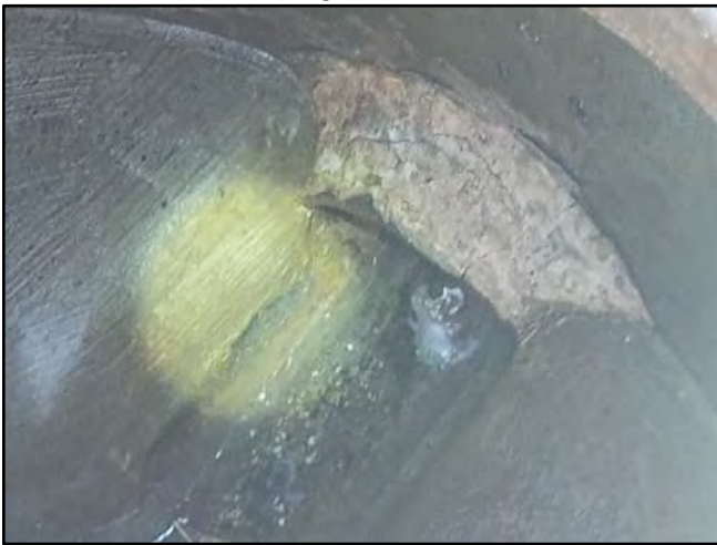
Image 5 – South Effluent Connection
