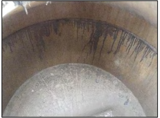
Image 4 – Cone/Base Joint
