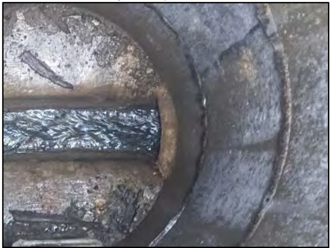
Image 6 – North Effluent Connection
