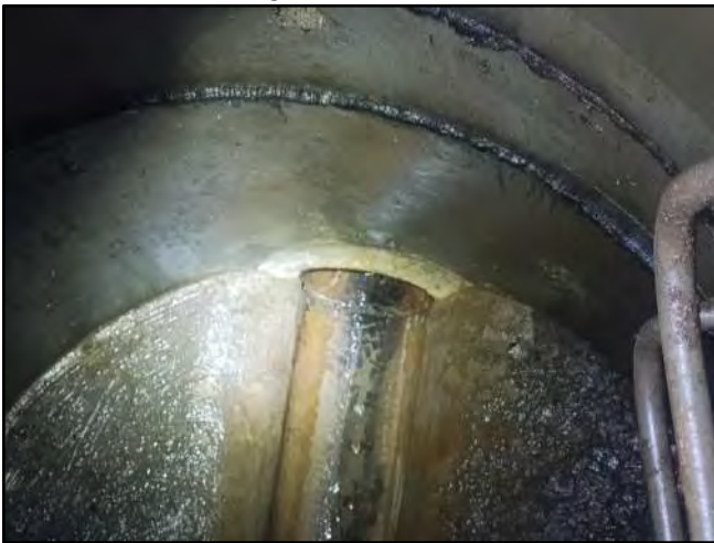
Image 5 – West Effluent Connection
