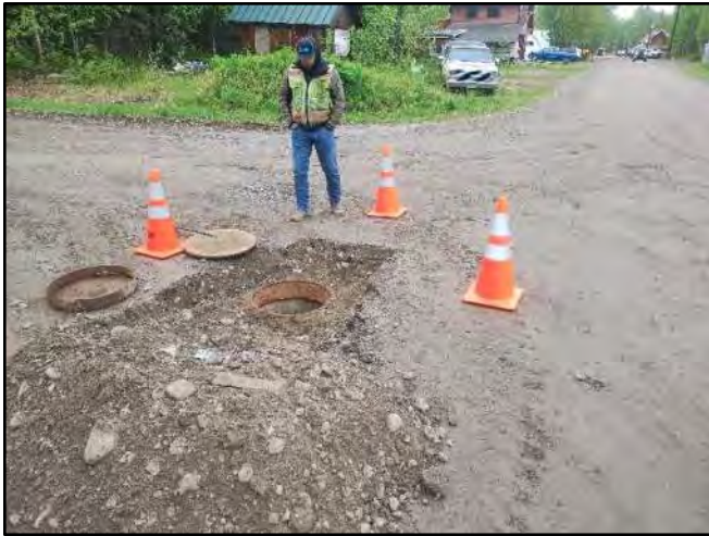
Image 1 – MH facing North along C St
