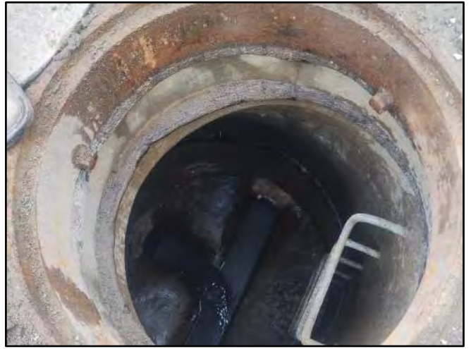
Image 2 – Frame and Chimney
