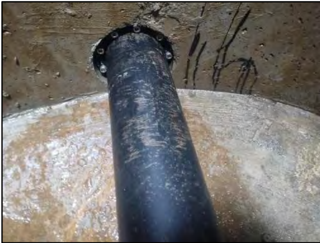
Image 3 – PVC Connection Link Seal
