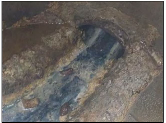
Image 4 – North Influent Connection
