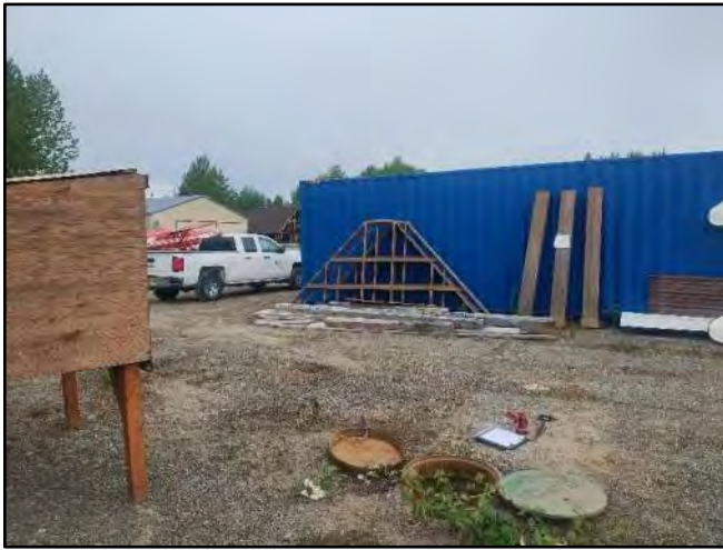
Image 1 – MH Facing North
