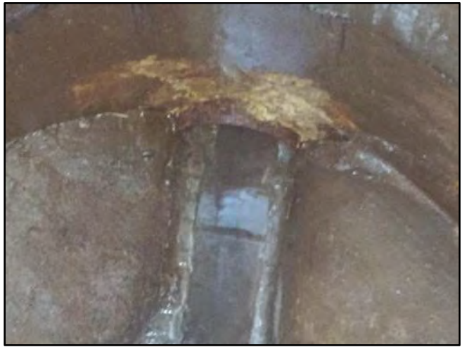
Image 4 – East Influent Connection
