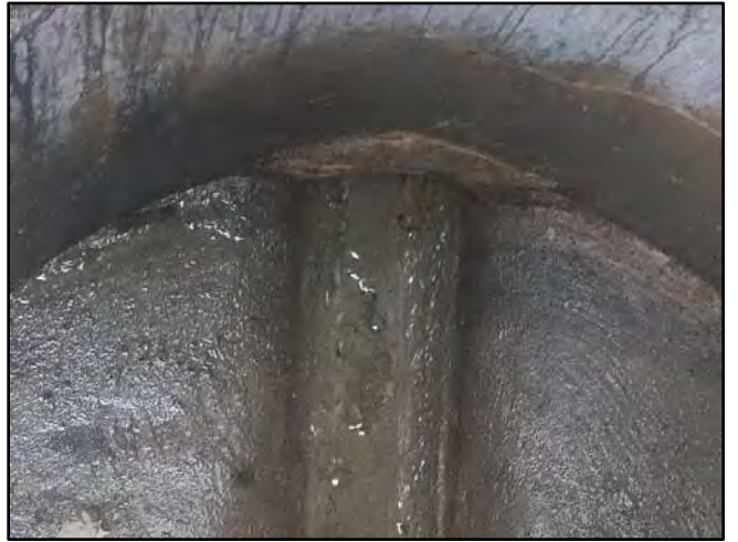
Image 4 – West Effluent Connection
