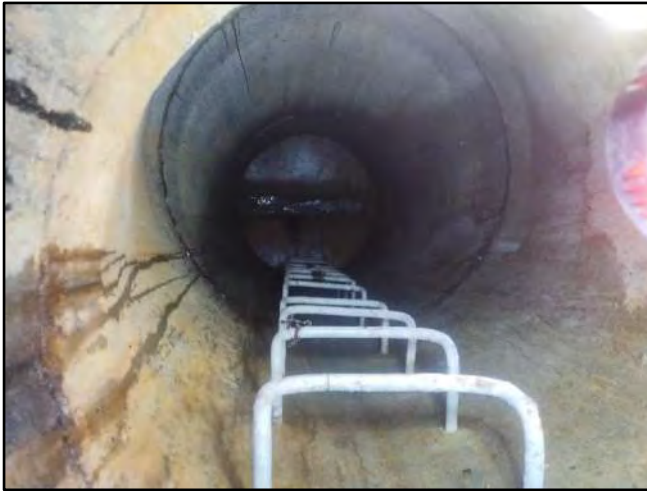
Image 3 – Chimney, Cone, and Stairs
