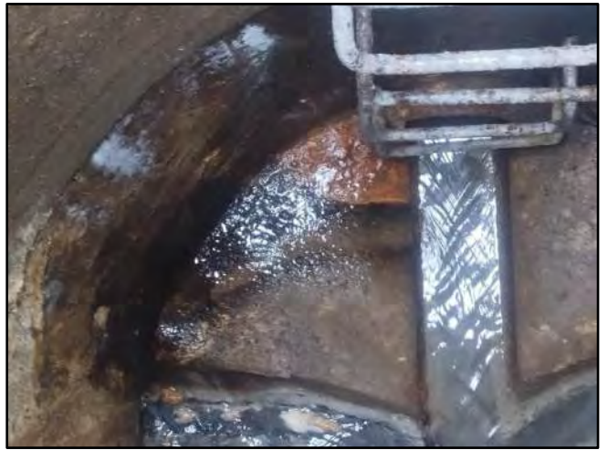
Image 4 – Northeast I&I Runner / Dripper
