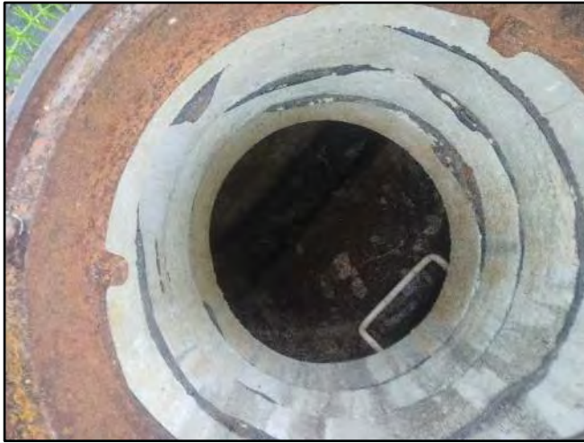
Image 3 – Frame and Chimney
