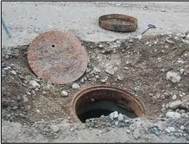
Image 3 – Cover, Catchpan, and Frame
