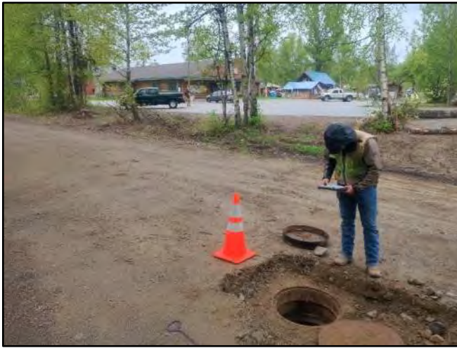
Image 1 – MH facing North towards Post Office
