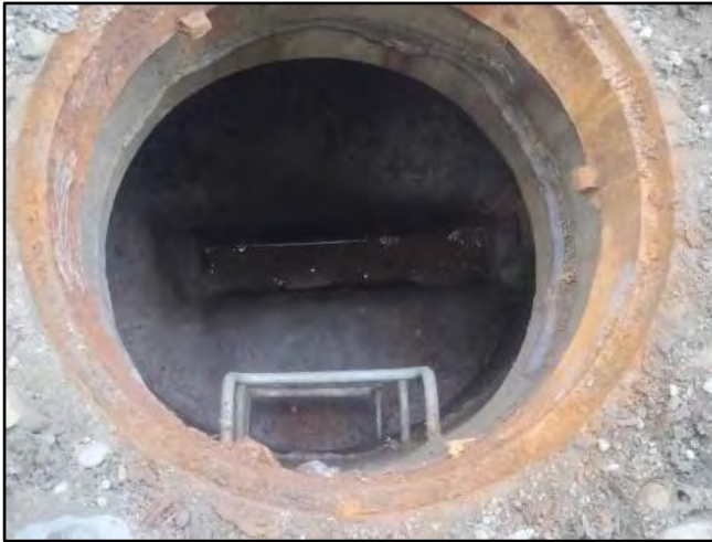
Image 3 – Frame and Chimney
