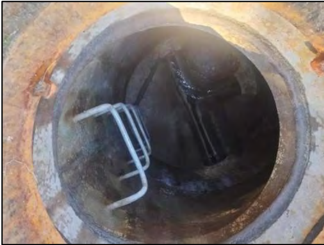
Image 3 – Frame, Chimney, and Cone
