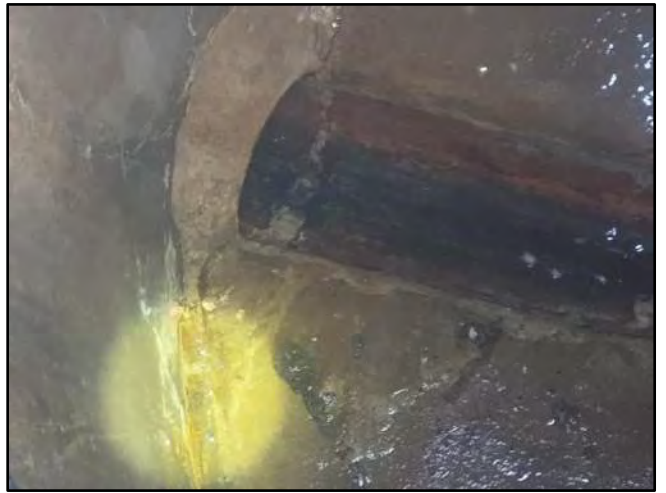
Image 4 – West Effluent Connection and I&I Dripper
