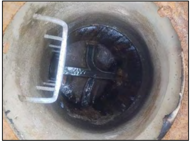
Image 2 – Frame, Cone, and Base
