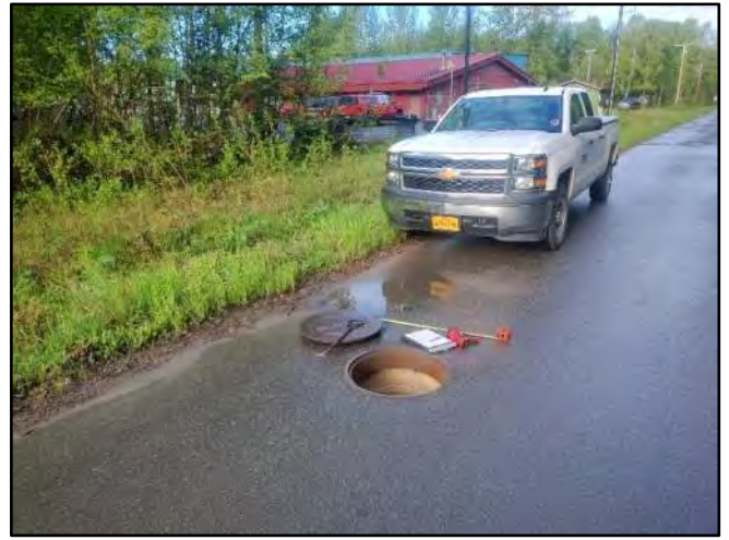
Image 2 – MH Facing Towards Fire Station
