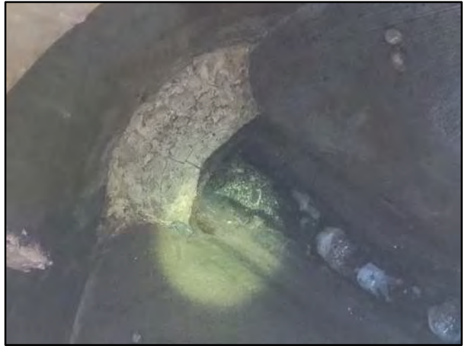
Image 4 – East Influent Connection
