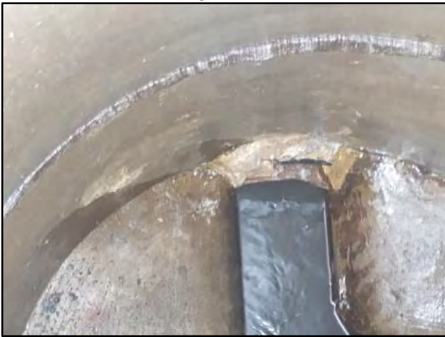
Image 5 – South Effluent Connection
