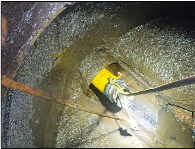
Image 5 – Southeast Influent Connection
