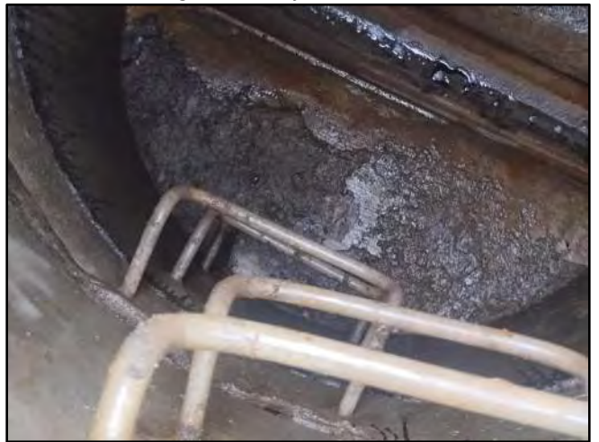
Image 6 – Solids Build-up on North Shelf
