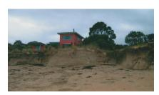
The District Plan's Current and Future Coastal Erosion Lines are available for this location and show that the properties seaward of SH25 are at risk from erosion; see photo from July 2008 storm. Push-ups helped to restore the dune in this location.
